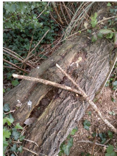
30. Deep crack in shed limb of T17.
